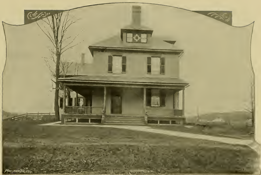
RESIDENCE OF CICERO GEARHART, ESQ., STROUDSBURG, PA.
